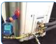
Vacuum with VG64-LX digital gauge
